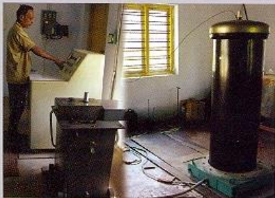
High Voltage Electrical Testing Machine upto 120KV
